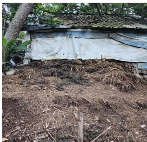
Figure 2. Condition of the cowshed
